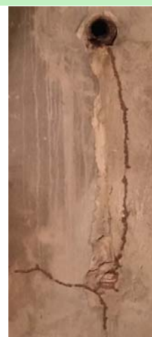
Inspect around the home for mud tubes that connect underground nest with your home
